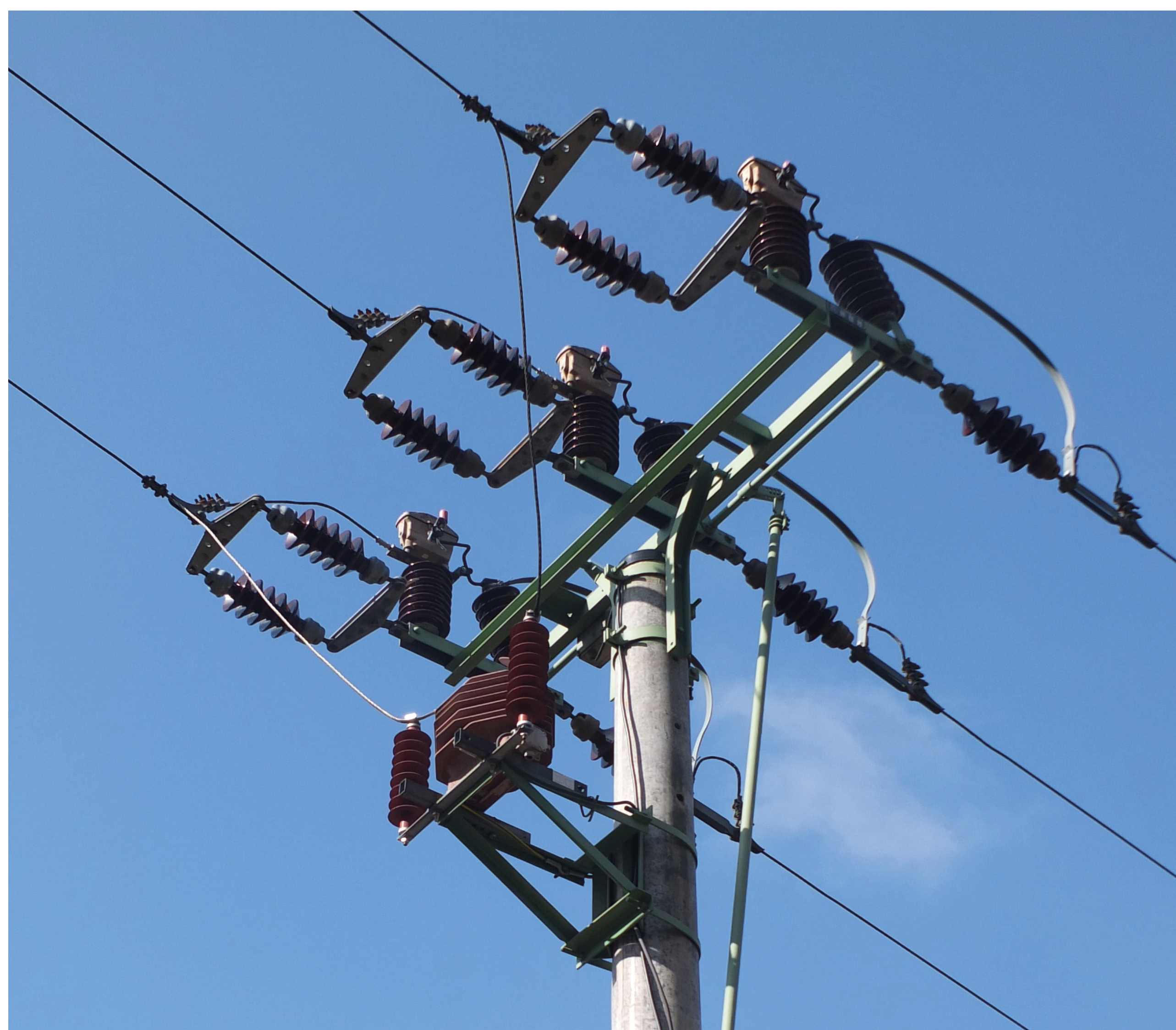
Remotely controlled switch – detail
