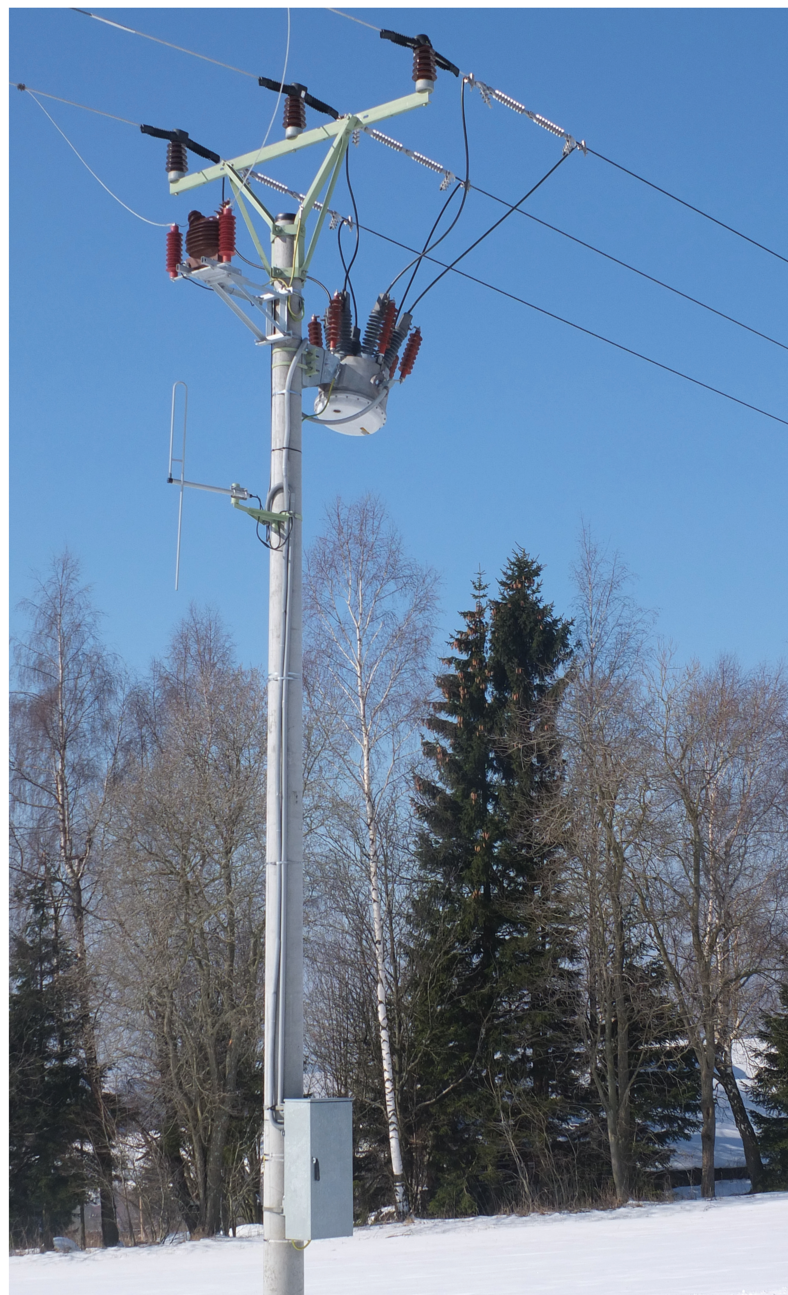
Recloser on a high-voltage pole
